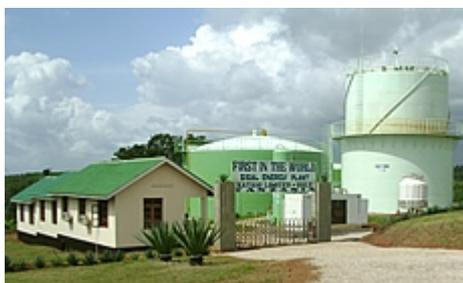
The Hale biogas plant uses sisal waste to produce electricity.
